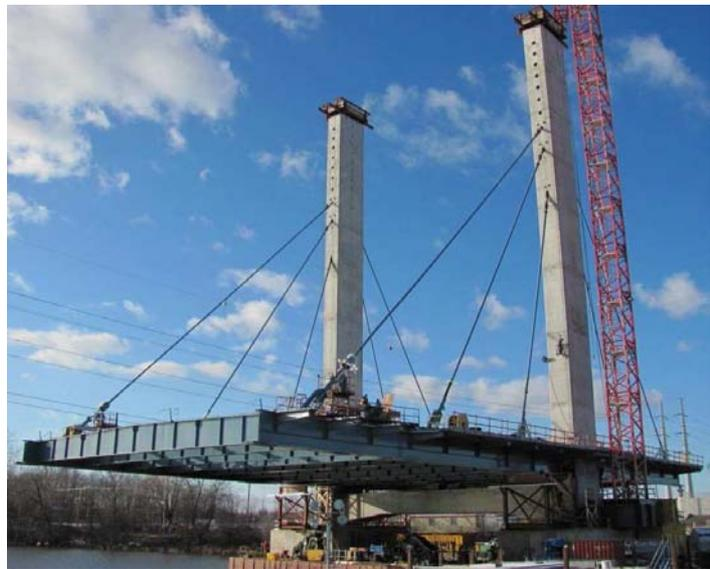
Figure 1- Cantilever Construction of Cable Stayed Spans.
