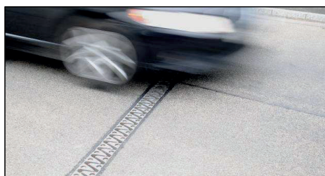
Fig. 1: Small movement expansion joint (single gap joint with noise-reducing surface plates)
